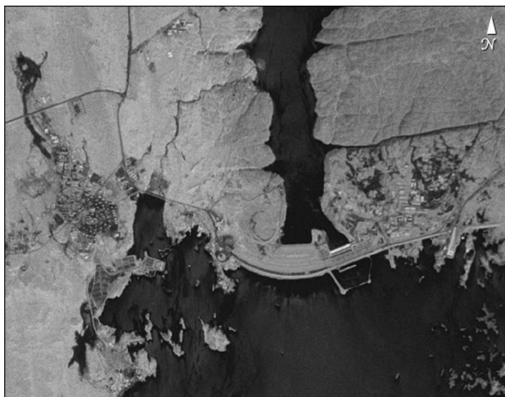
Fig. 1. Location of the High Dam and the High Dam Lake (NASA satellite photo)
