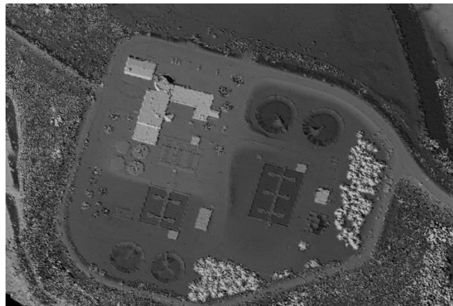
Picture 2 – 150 kHz LIDAR image of water treatment plant at 1250 meters demonstrates MPiA technology
